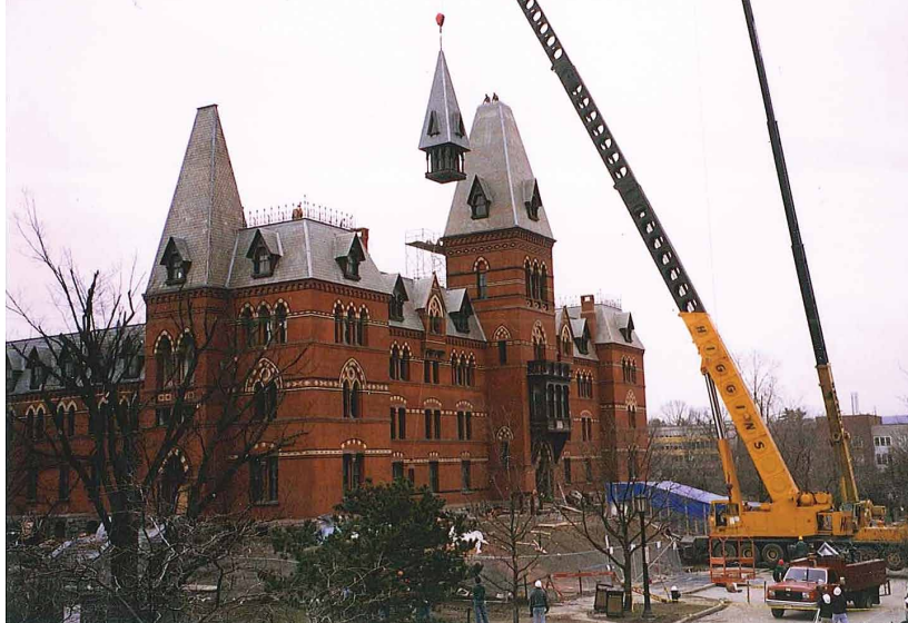
→ Re-crowned: Sage Hall's spire was reconstructed on the ground from old photographs, researched by the architect and by Cornell, and hoisted into place atop the building's west tower on March 3, 1998. Cornell's sheet metal shop replicated a unique weather finial from old photographs to preserve the building's historical integrity.
